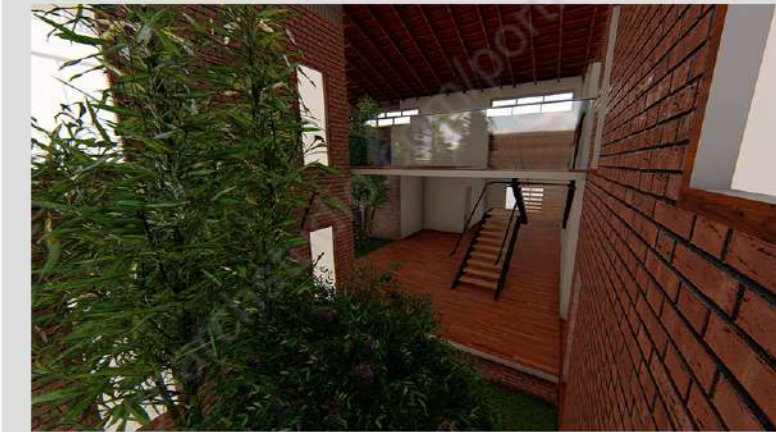
VIEW FROM THE COURTYARD TO THE INTERIOR.
