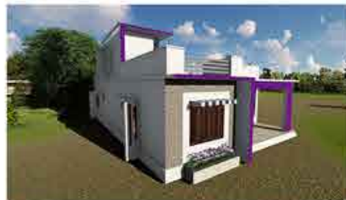
On going outside work
