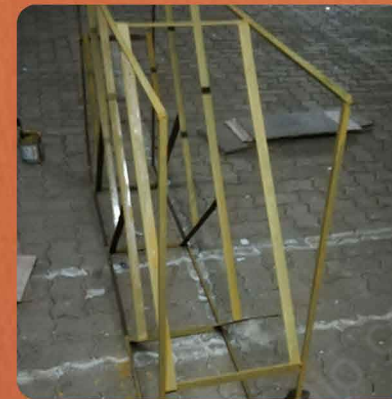
THE ENTIRE FRAME WAS COATED WITH METAL PRIMER
